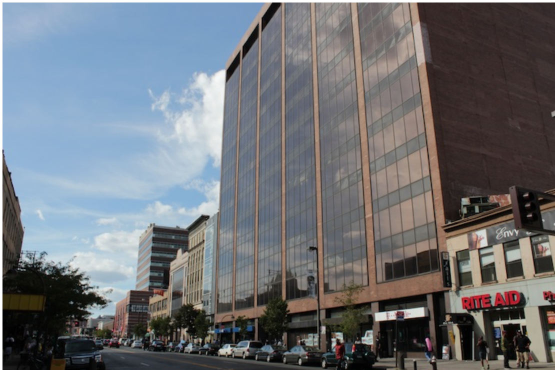
Fig. 24 – Bill Clinton's office building.
