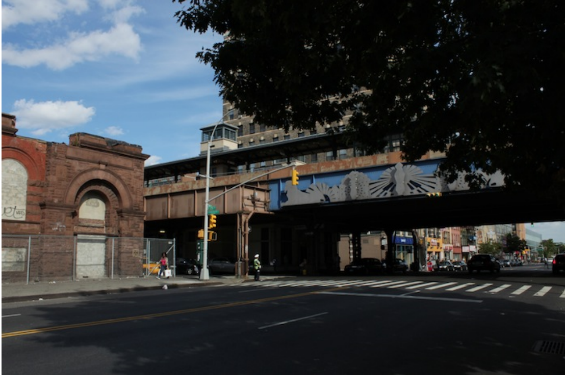
Fig. 31 – The 4, 5, 6 Subway Bridge, 125 th Street station.
