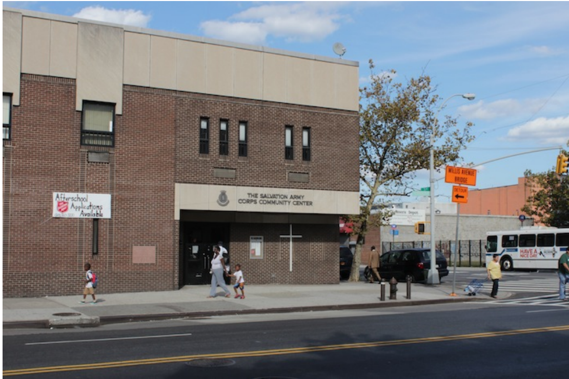
Fig. 35 – The Salvation Army Corps Community Center, 3 rd Avenue.
