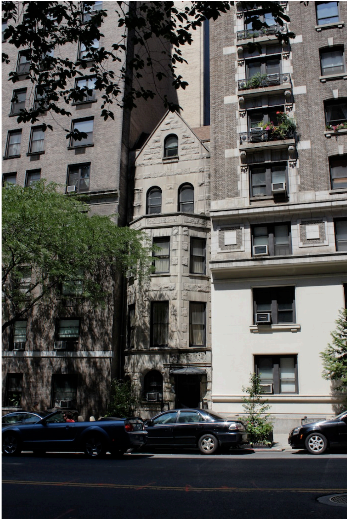
13 – Mediaeval structure trapped between two high-rises.
