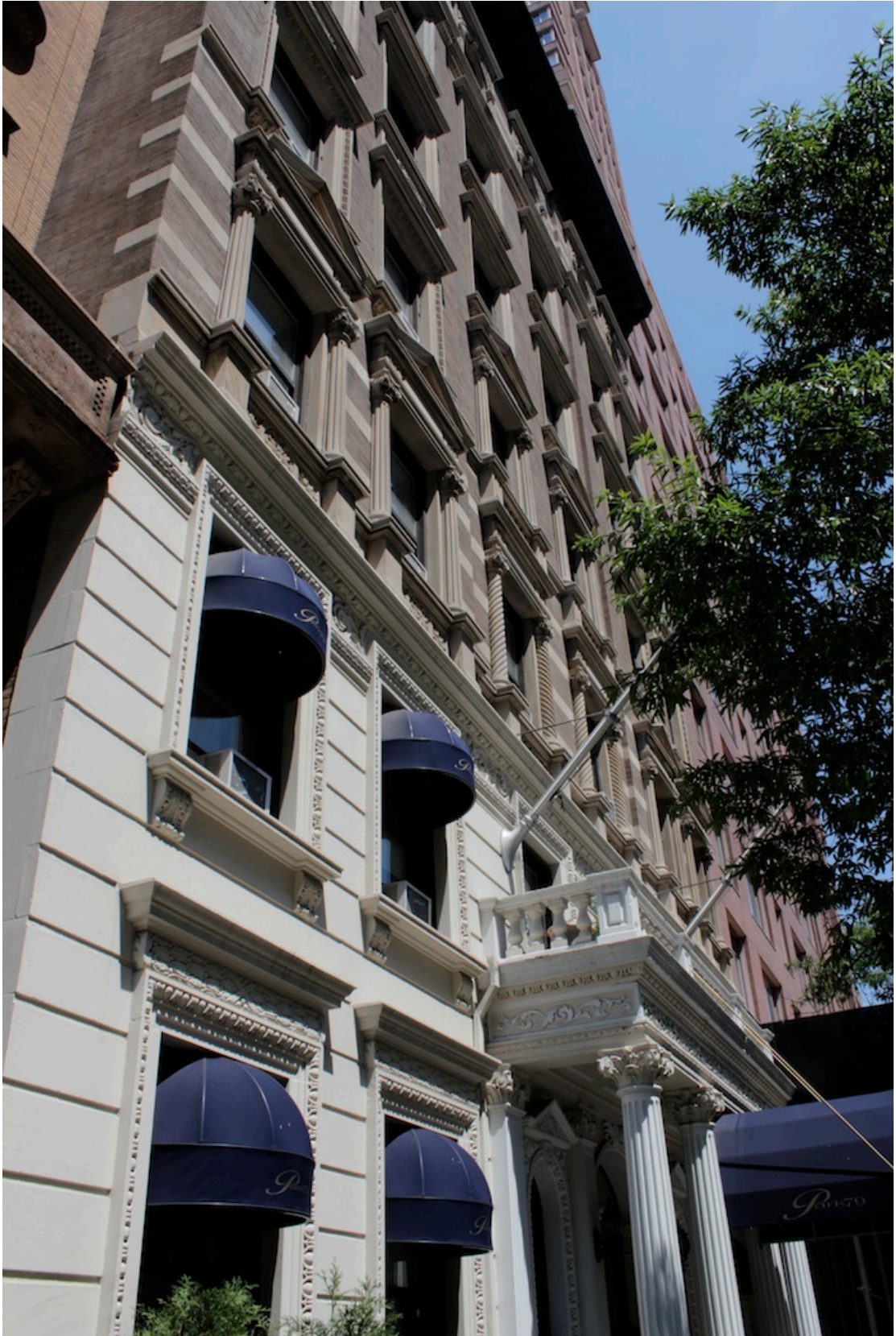
18 – Another modern, upscale apartment block.
