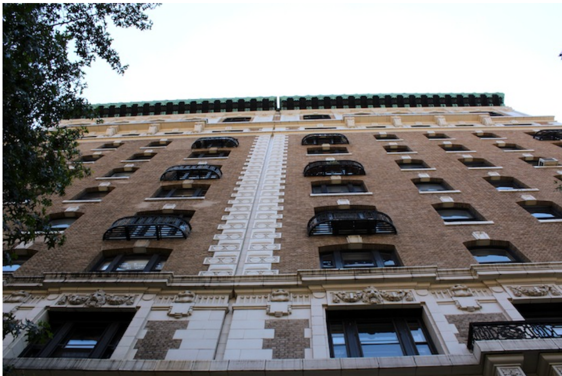
6 – Beaux-Arts detailing on the façade of another waterfront property.
