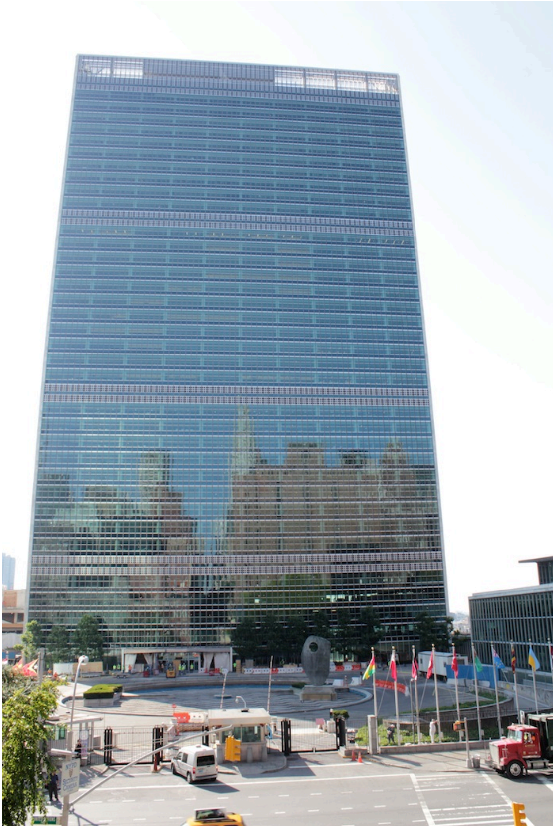
1 – The United Nations Secretariat Tower, completed in 1952 and designed by an international committee of architects, including Le Corbusier, Oscar Niemeyer, amongst others.
