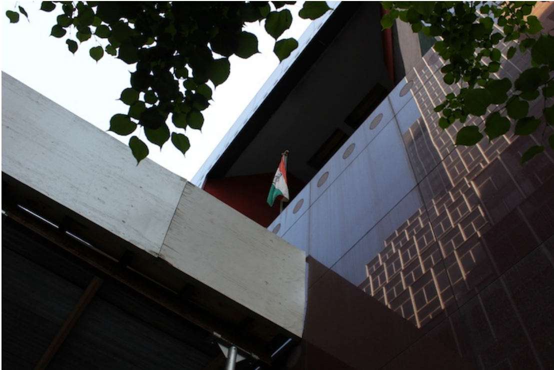
10 – No. 245: The Permanent Mission of India to the United Nations (1991), designed by Indian architect Charles Correa. The Pfizer Building, just across the street, is reflected on the building's façade.
