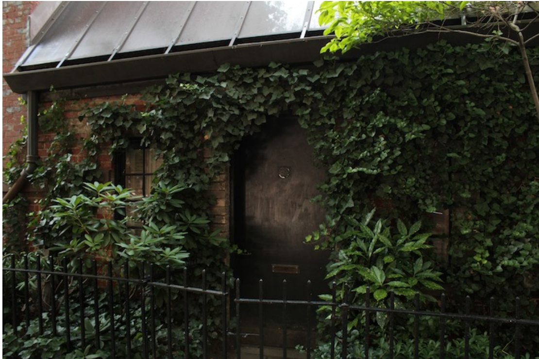
47 – A quaint little cottage-like structure possibly marks the entrance to the Bleecker Street Gardens .
