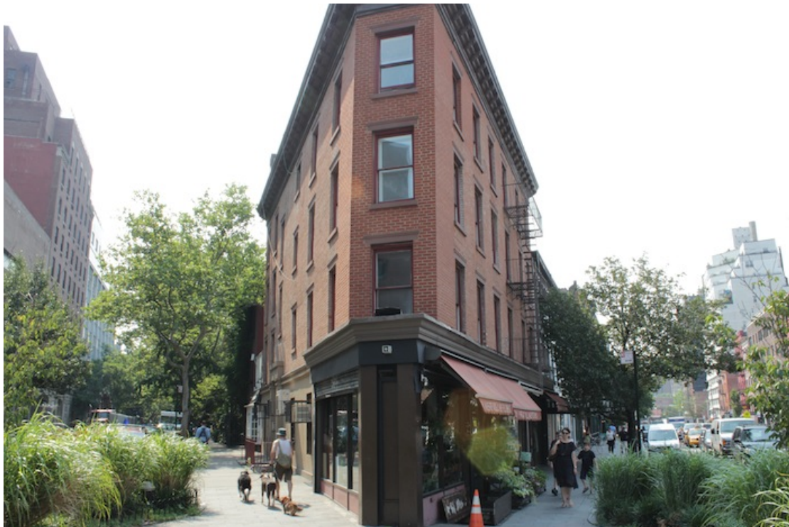
39 – A triangular building flanked by 11 th St and Greenwich Ave. It looks like a barrier separating the souls of the living from the dead. It also marks the end of 11 th Street's straightforward path.
