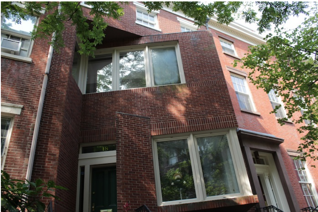
33 – No. 18: The Weatherman House , originally built in 1845, and rebuilt in the modernist style in 1978, after a bomb blew up here.
