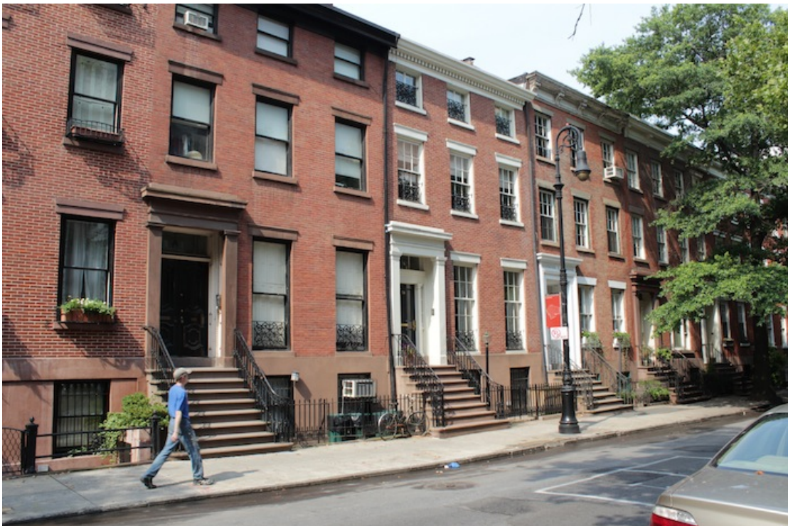
35 - Squeaky-clean restored facades in the Greenwich Village Historic District , channeling Disney.
