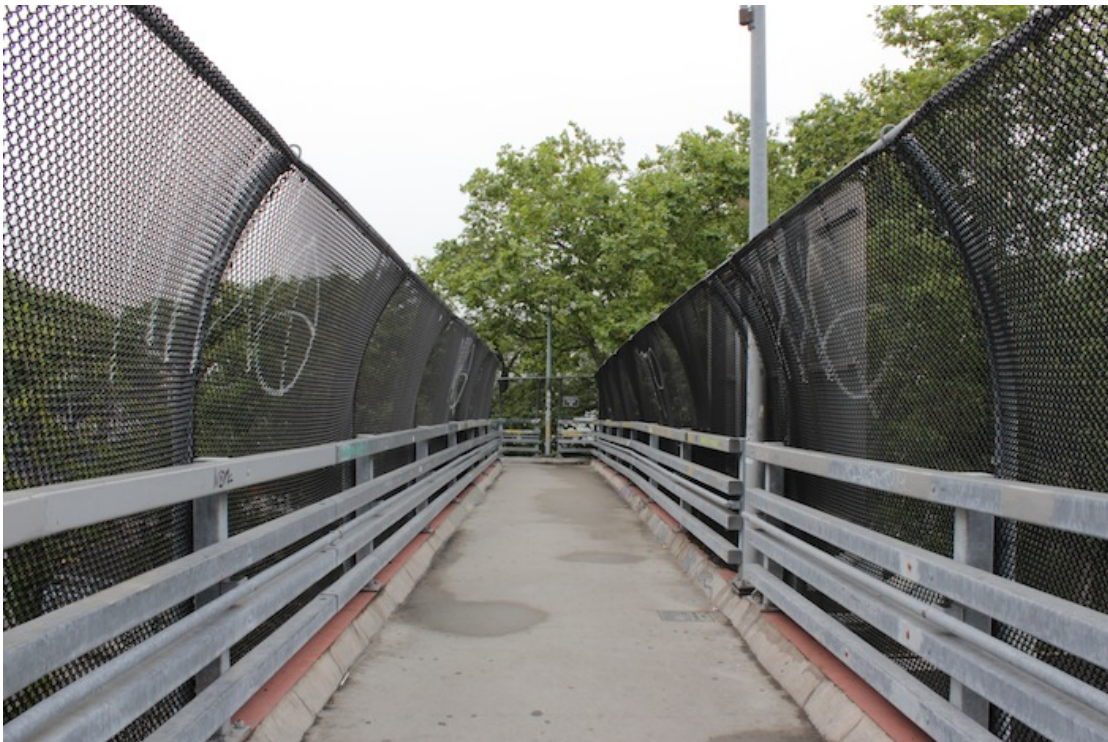
2 – Cast beyond the open gates of heaven: the footbridge across FDR Drive.
