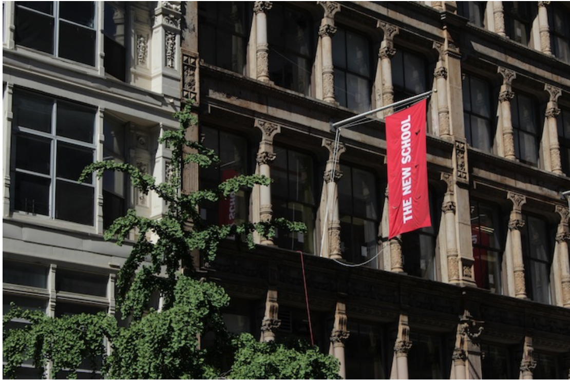
29 – Offices of The New School, housed in an 1880 cast-iron clad building by D. & J. Jardine. It used to be a retail store.
